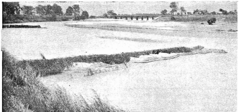
ONE OF THE GROYNES—A PROJECTION of earth and stone—with accumulation of siltation after flooding; also, in the foreground, growth of willow and grass along the bank. Pilot channel on the right.
